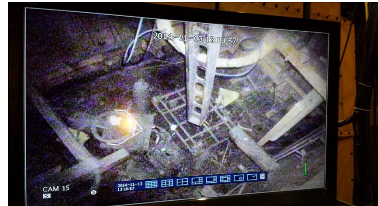
Extraction Cell-1 Before Deactivation
