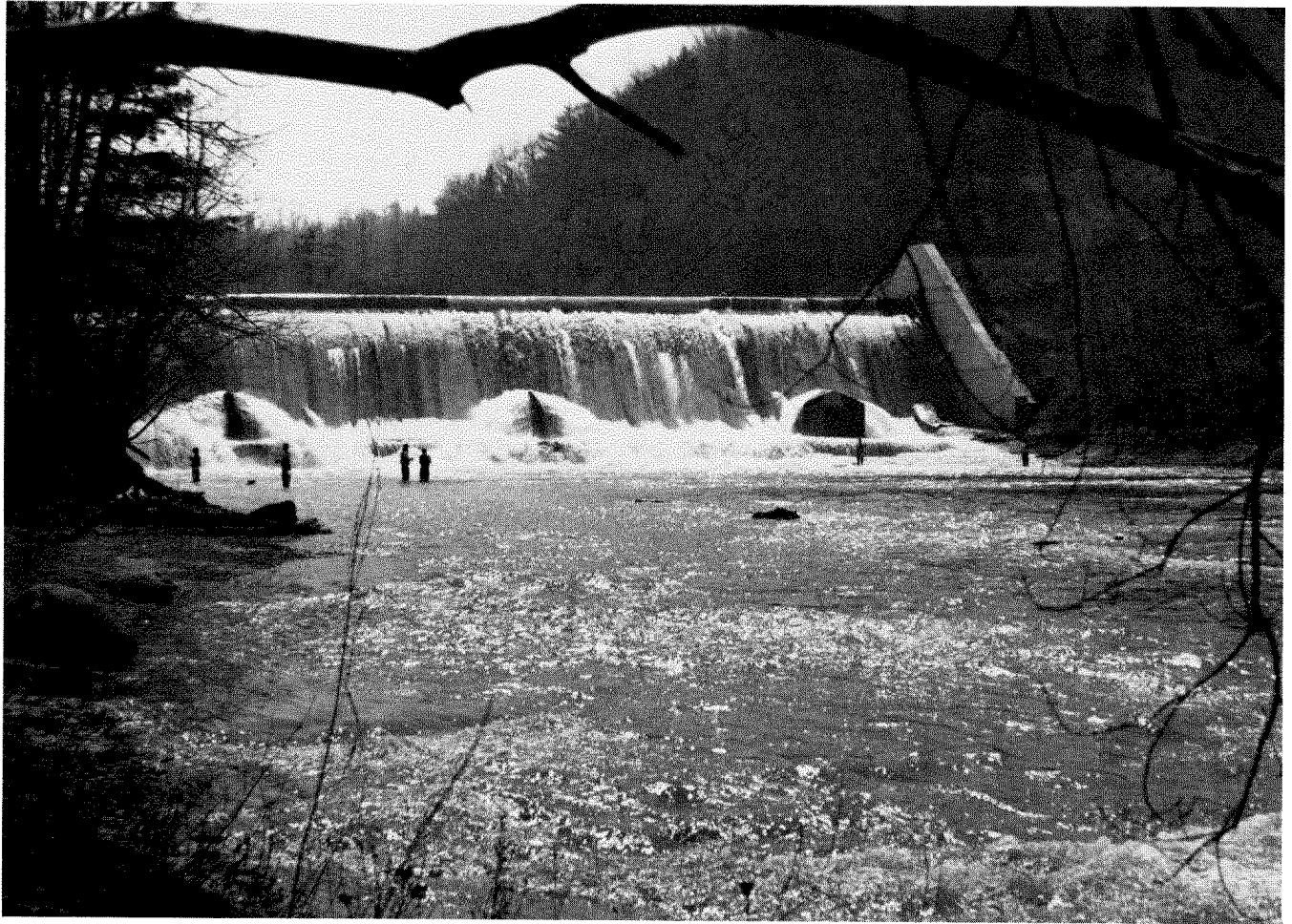
Springville Dam on Cattaraugus Creek
