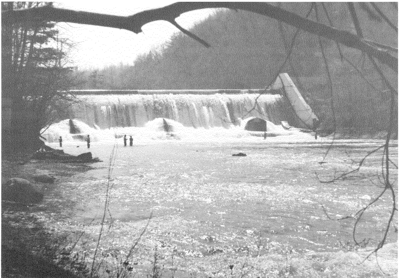
Springville Dam on Cattaraugus Creek
