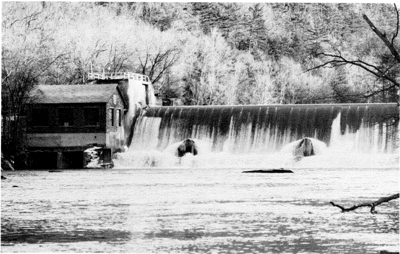
Springville Dam on Cattaraugus Creek
