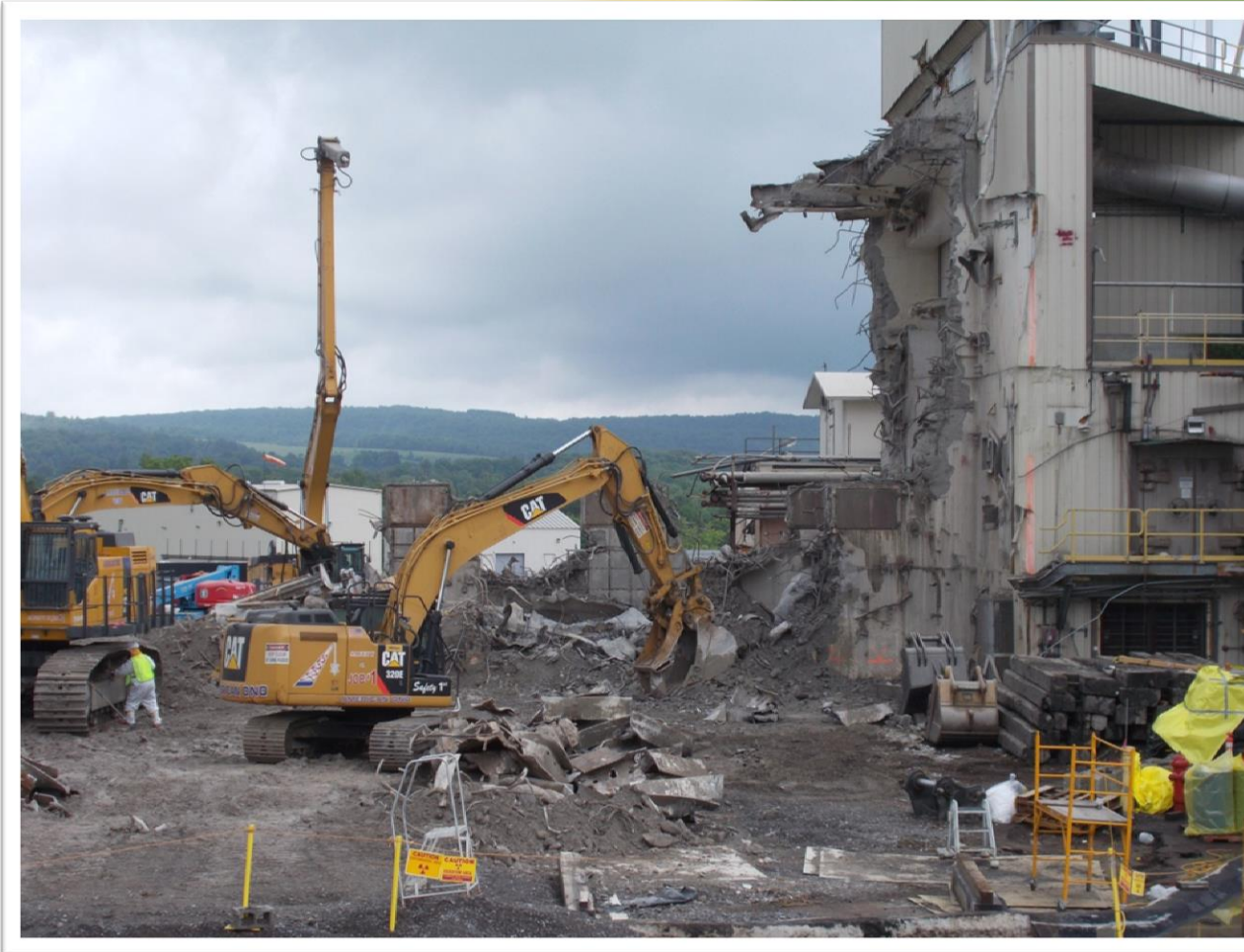
Vitrification Facility Demolition, June 13 Excavator preparing demolition debris for loading
