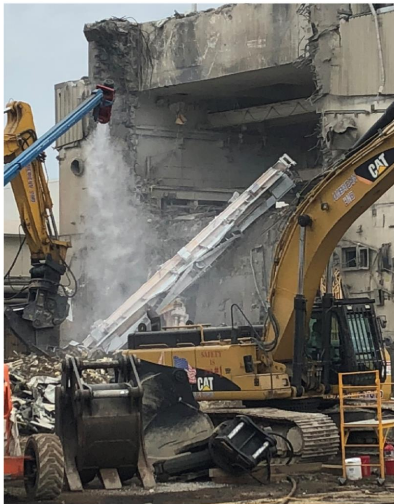
Vitrification Demolition, August 13, 2018 Crews remove VIT process cranes
