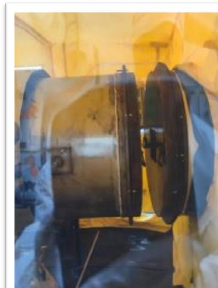
VEC 36-inch duct separation cuts
