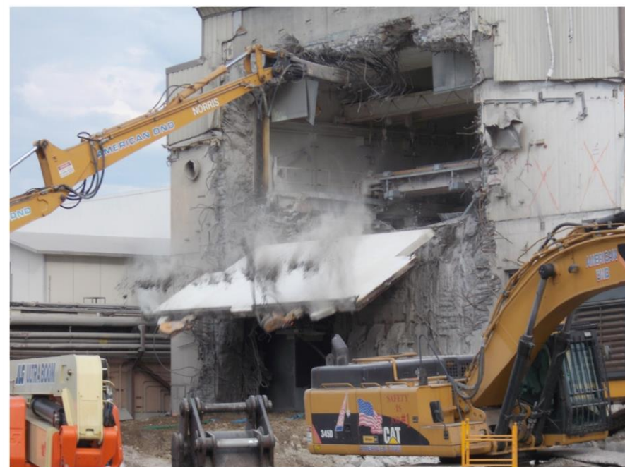
Removal of 100-ton Crane Maintenance Room Shield Door
