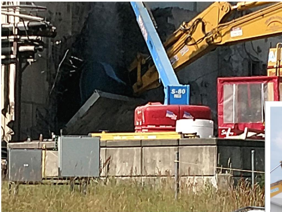
Removal of 60-ton Transfer Tunnel Shield Door
