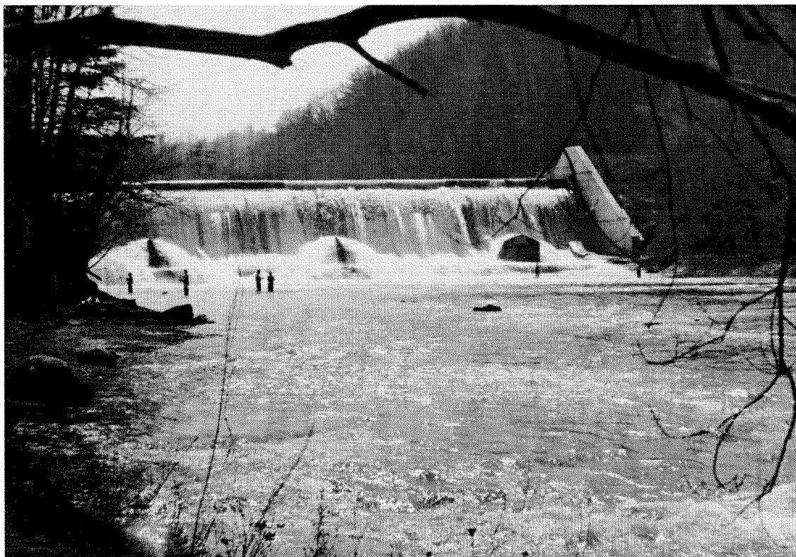
Springville Dam on Cattaraugus Creek
